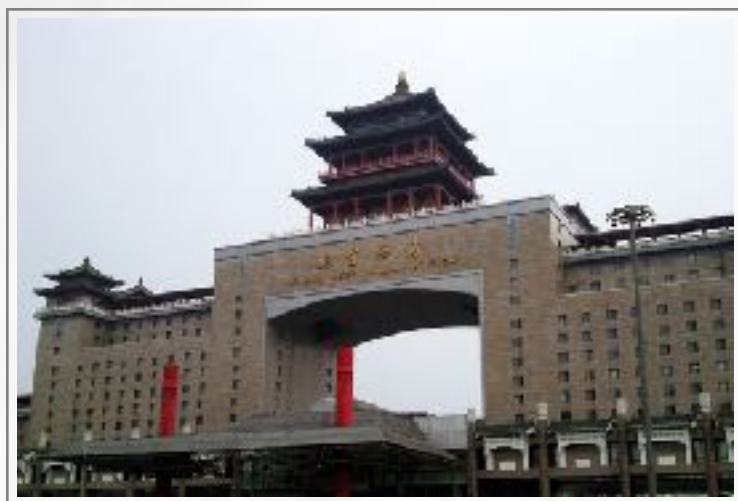
图片 3大屋顶风格：北京西站，1996. https://upload.wikimedia.org/wikipedia/commons/c/cf/North_house_of_Beijing_West_Railway_Station.jpg
